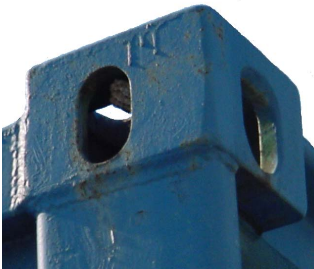
Figure 4. Corner Fitting
