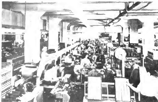
The process of cigarette making, packaging, and placing the packs in cartons ready for the consumer.
